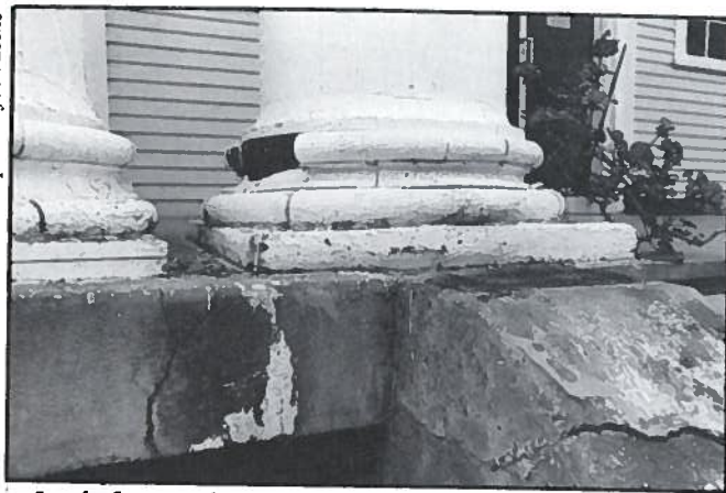
Look for cracks in the foundation that indicate movement, possibly breaking up base parts between the joints.
